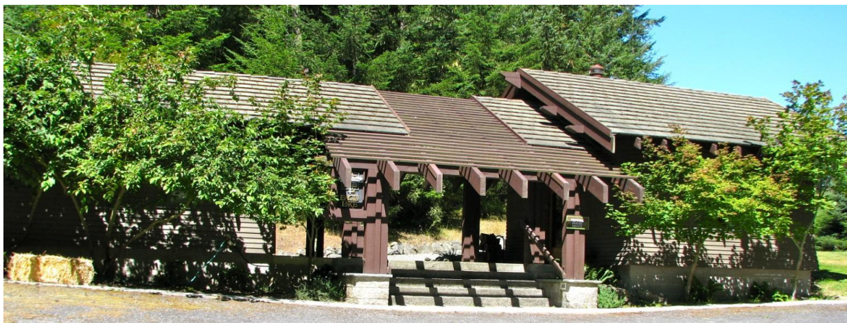
Figure 2 The meeting house is an example of using traditional architecture with shallow pitched roofs, broad deep eaves, long horizontal lines, and wood exterior finishes
